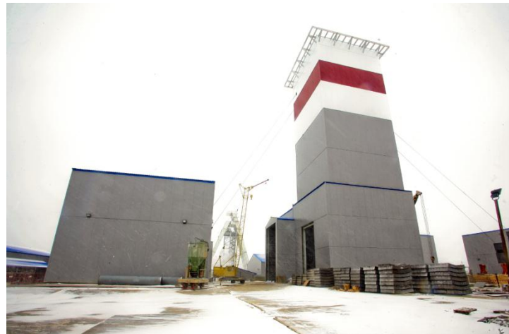
Cage shaft construction site*
