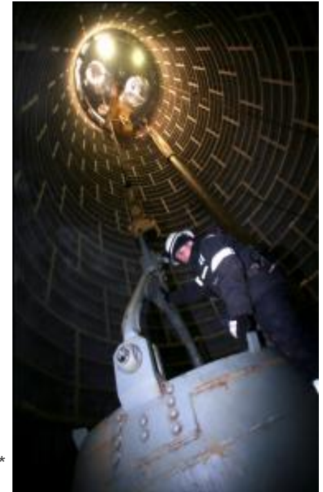
Skip shaft sinking*
