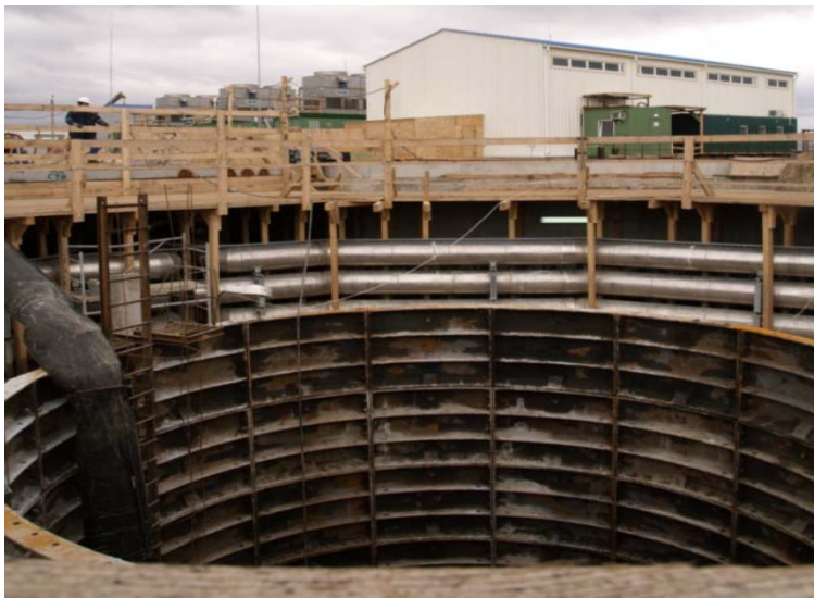
Skip shaft pre-sink
