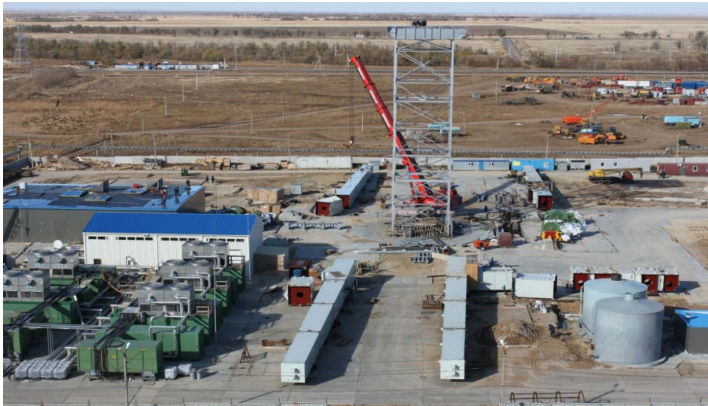
Skip shaft construction site and cooling system
