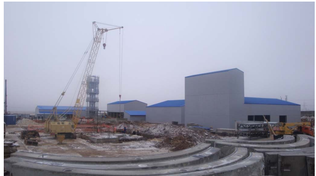
Cage shaft construction site
